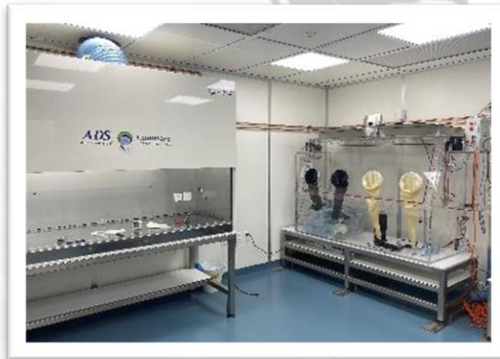
Lawrence, Massachusetts (Operational – Producing Generators)
